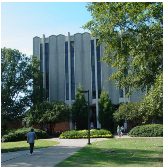
Figure 8 Example for a building constructed using concrete - Allen Hall at MSU
